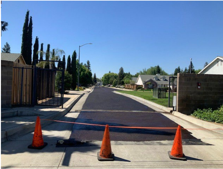
Slurry Seal Work June 2022
