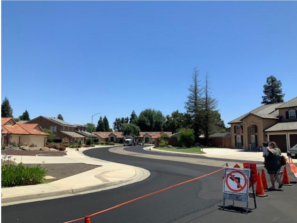
Slurry Seal Work June 2022
